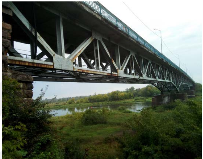
Bridge over the Berezina River at 230,961 km of the P-43 road
